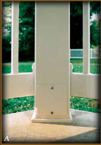
Column detail with heavy duty railing attachment
