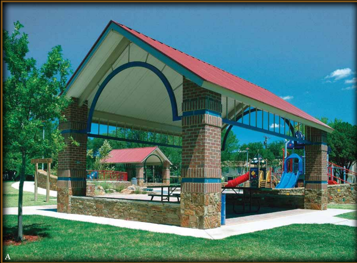
Rose Meadows Park, Irving, TX: While uncomplicated in design, the Orlando model has been one of our most popular to customize, as shown on these handsome 20' x 28' models. CRS created curved ornamentation from the designer's working drawings. The brick and stone work is by others. Shown with Bright Red R-panel roof and T & G subroof.
