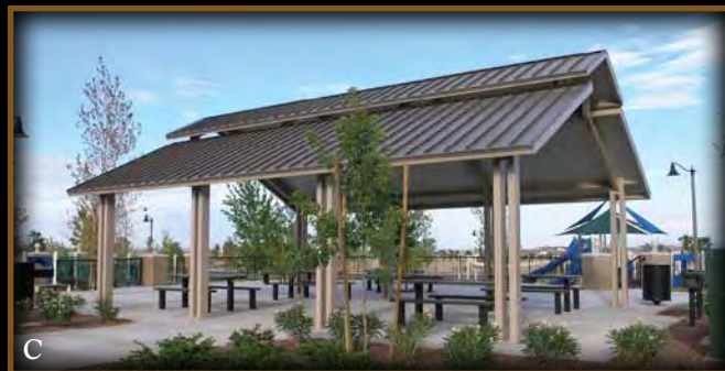
C Walton Park, Verrado, AZ: 26' x 34' Cheyenne model with 12" o.c. standing seam steel roof in "Weathered Copper" color. Features double tube steel columns with rafter extensions.
