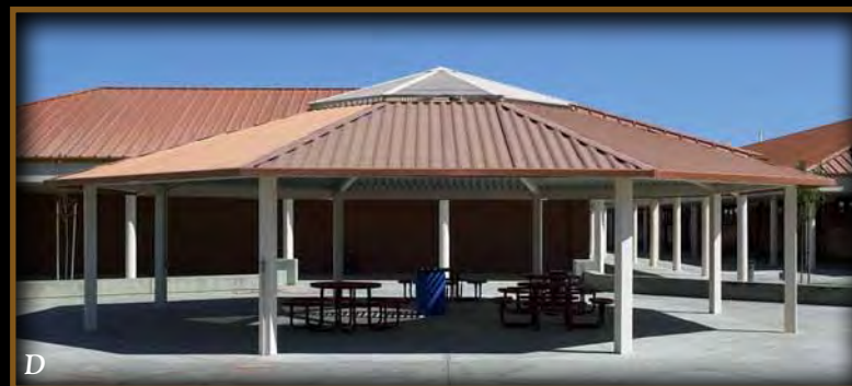
Weston Ranch HS, CA: A 2" x 2" lattice tube 2nd tier allows light and air movement on this 41' model. Metallic Copper HR-36 roof matches buildings. CA DSA approved.
