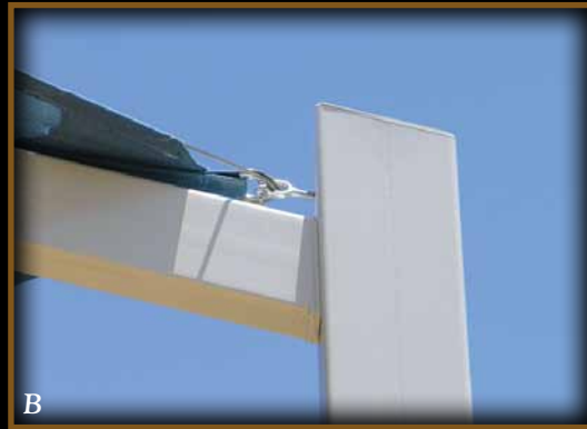
Mehl Family Foothills Park, Tucson, AZ: 48' hexagon showing "Coolaroo" fabric to post connection detail.
