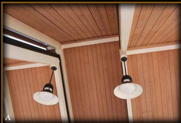
Ceiling Detail: Select 2" x 6" T & G sub-roof w/ lights & hidden wire runs.
