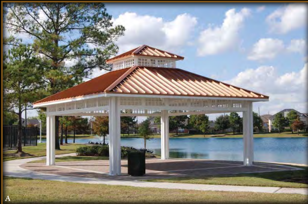
Barker Lake, Houston, TX: 25' x 25' Scottsdale, with cool Copper Penny 12" o.c. standing seam roof with Traffic White powder coated frame, custom lattice ornamentation and cluster columns.
