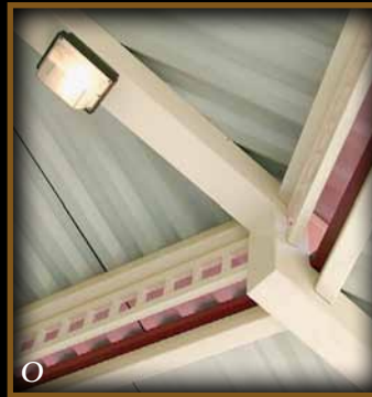
Optional H.D. picket ornamentation, 1" pickets 5" o.c with concealed wiring for lighting. Cut & mitered main beam
