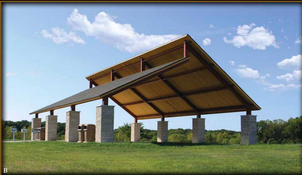
Forest Preserve, Batavia, IL: 36' x 50' Northwest model with 2" x 6" T & G sub-roof and fascia with shingles. Stone surrounds by others.
