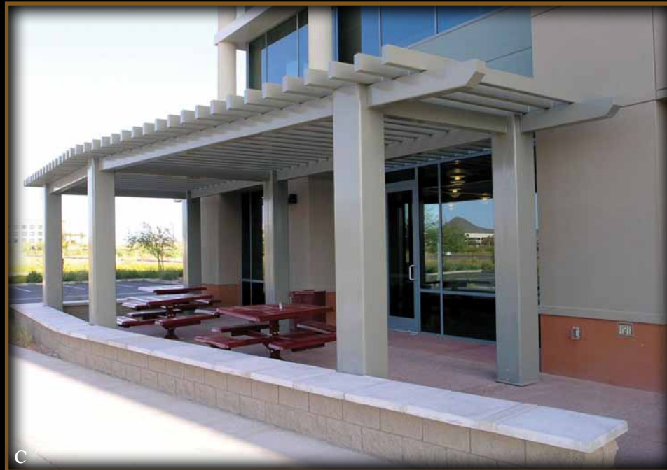
C Arizona State Credit Union, Phoenix, AZ: This 18' x 40' H.D. Trellis compliments the clean massive lines of the adjacent building providing a shaded area for employee breaks.
