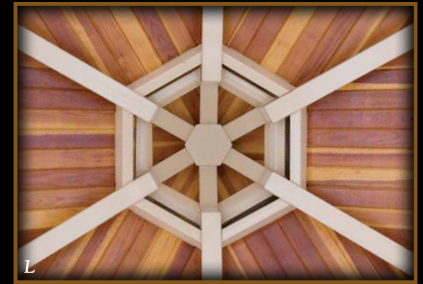
Custom cedar 2" x 6" T&G detail on Dallas model with cupola.
