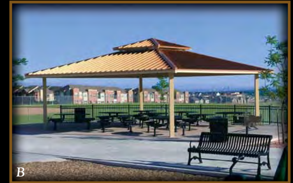
Ridgeway Community Park, Lone Tree, CO: 30' x 30' Scottsdale model with 12" o.c. standing seam steel roof in Copper Penny color.
