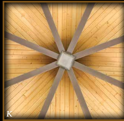
Standard tongue & groove and lighting detail.
