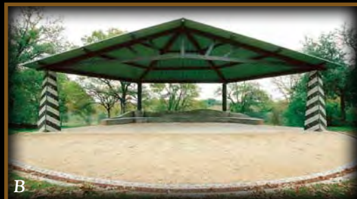
B Community Park, Austin, TX: This 45' model features R-panel roof with tile mosaic columns by Twyla Arthur.
