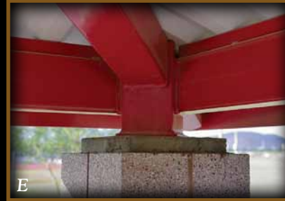
Denver column connection detail
